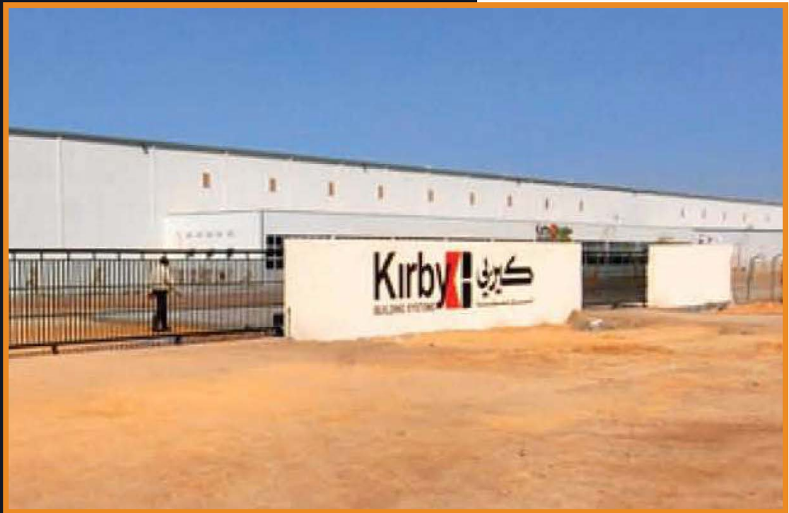
Location : Jazeera Client : Kirby Building Systems
